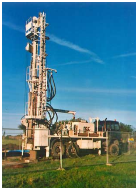
Typical borehole drilling rig
