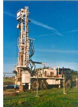
Typical borehole drilling rig
